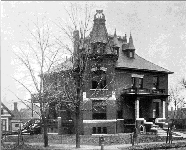
103 West Wood Street
